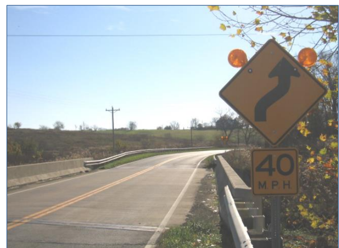
Figure 34. Flashing beacons on advisory curve sign (Vest et al. 2005)
