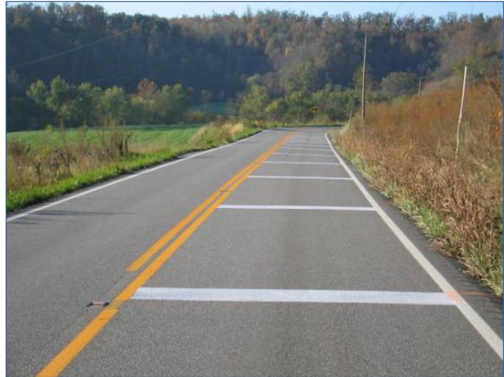
Figure 15. Equally-spaced transverse lines (Vest et al. 2005)
