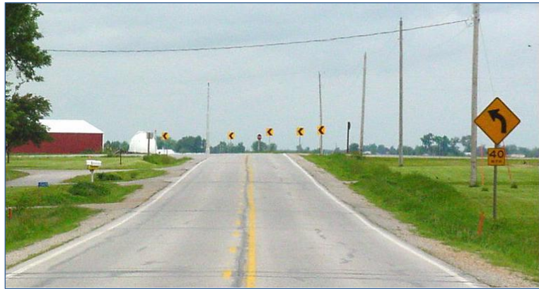
Figure 2. Oversized chevrons on US 6 in Johnson County, Iowa (Tom Welch, Iowa DOT)
