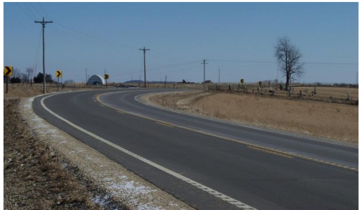
Figure 24. Edge-line and centerline rumble strips
