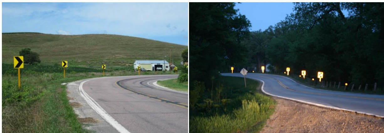
Figure 23. Reflective treatment added to existing chevron posts
