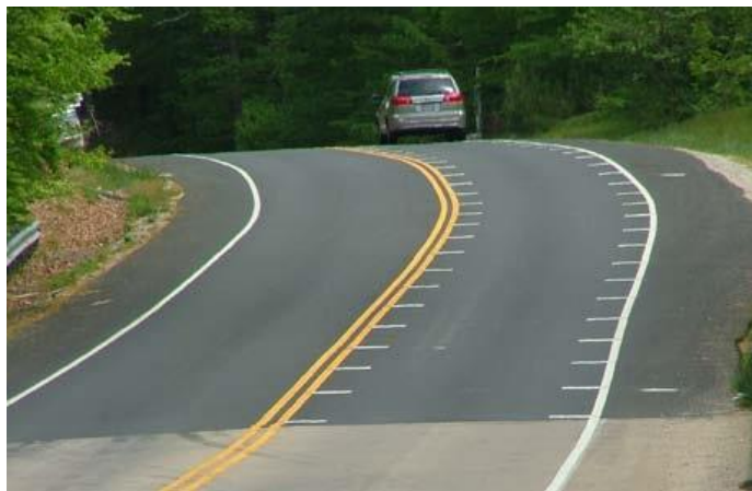
Figure 9. Optical speed bars (VDOT 2006)
