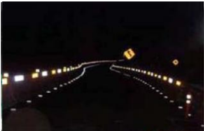
Figure 4. Nighttime view of retroreflective sheeting (McGee and Hanscom 2006)
