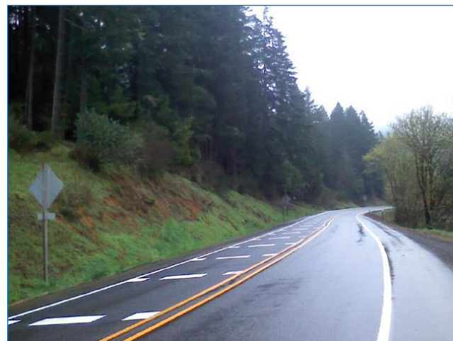
Figure 8. Various on-pavement curve markings
