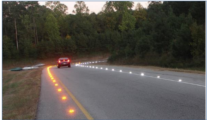
Figure 42. In-pavement lighting (FHWA 2011)
