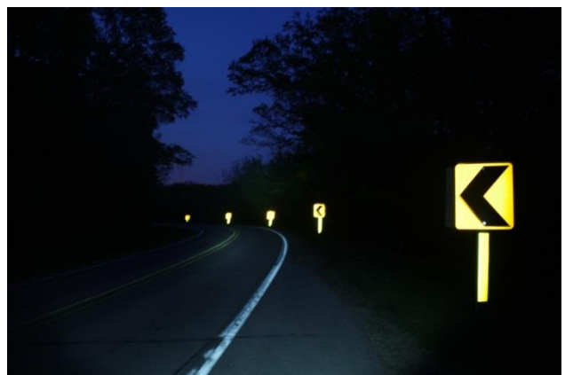
Figure 19. Retroreflective treatment on chevron posts day and night
