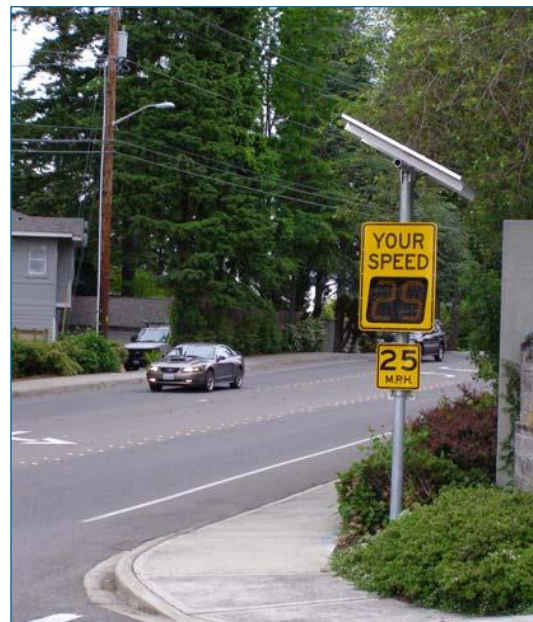
Figure 39. DSFS system in Bellevue, Washington (City of Bellevue 2009)
