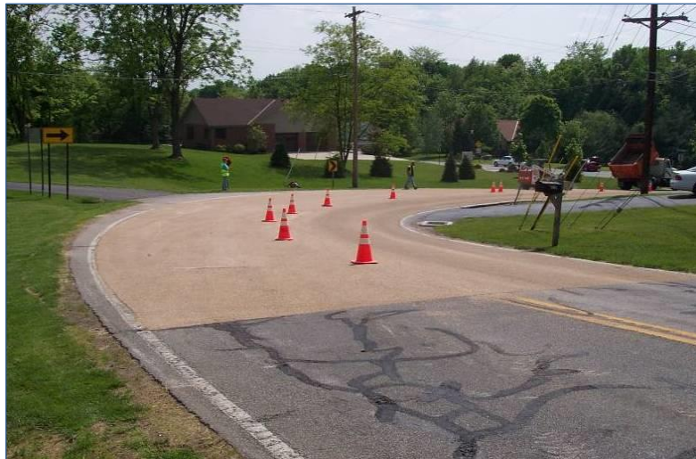
Figure 5. High-friction treatment (The Transtec Group, Inc., highfrictionroads.com )
