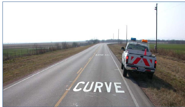
Figure 31. On-pavement curve markings (Chrysler and Schrock 2005)
