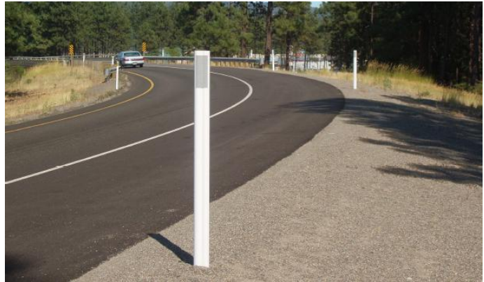
Figure 18. Delineator posts along a curve ( www.pexco.com/Pages/PexcoTrafficRDP.aspx )
