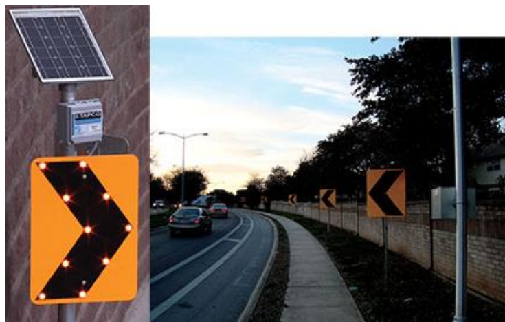
Figure 36. Sequential dynamic curve warning system (FHWA 2012)
