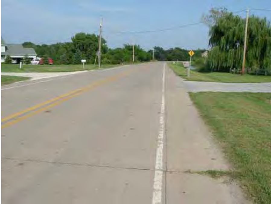
Figure 4. Paved shoulder with maintainable slopes
