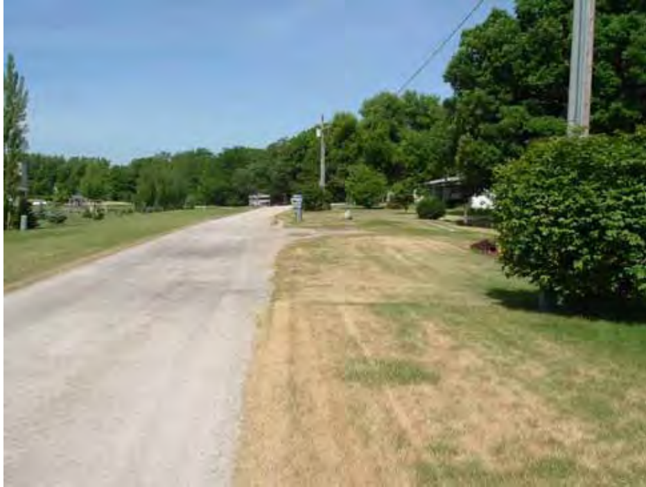
Figure 6. Unpaved local rural subdivision road
