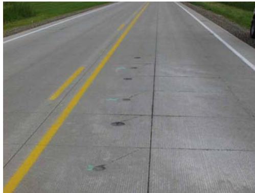
Figure 10. Temperature and strain gages along Iowa highway 13
