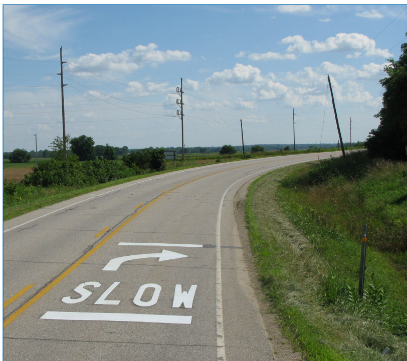
Supplementary on-pavement markings showing a curve arrow and a SLOW warning between two perpendicular bars were evaluated
