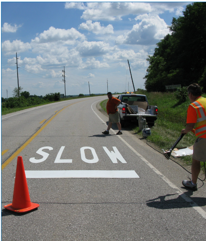
Installation of supplementary on-pavement markings on DMC 99
