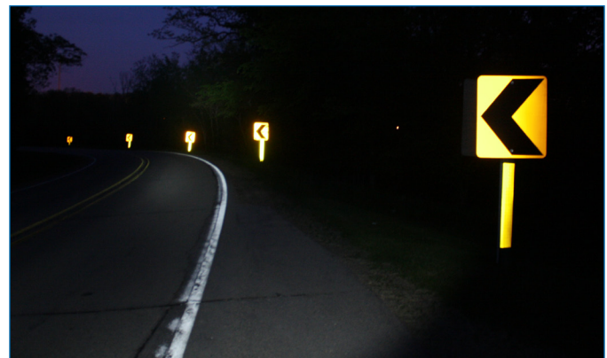
Retroreflective chevron post treatments on US 52 at night
