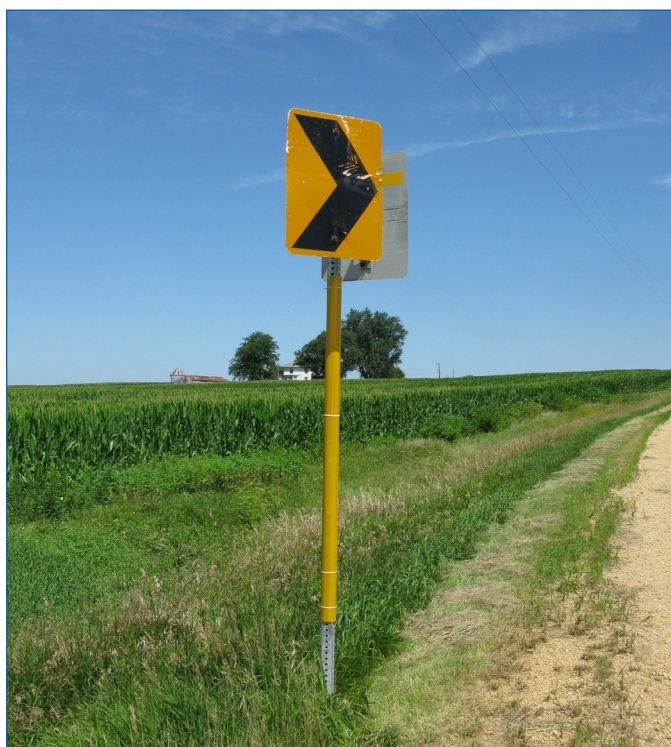
Supplementary post-mounted retroreflective material on County Road Y-52
