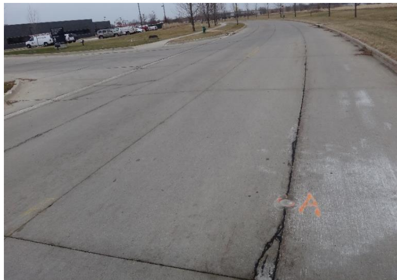
Figure 21. Field view of the location of Core 4, showing joint distress
