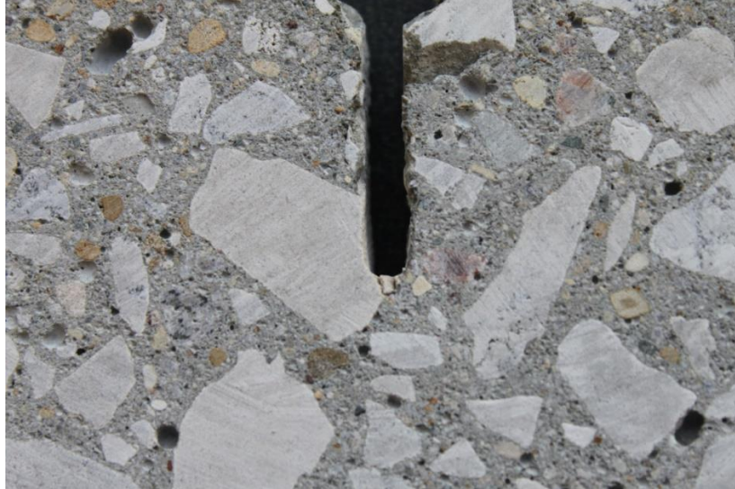
Figure 26. View of damage at saw cut tip
