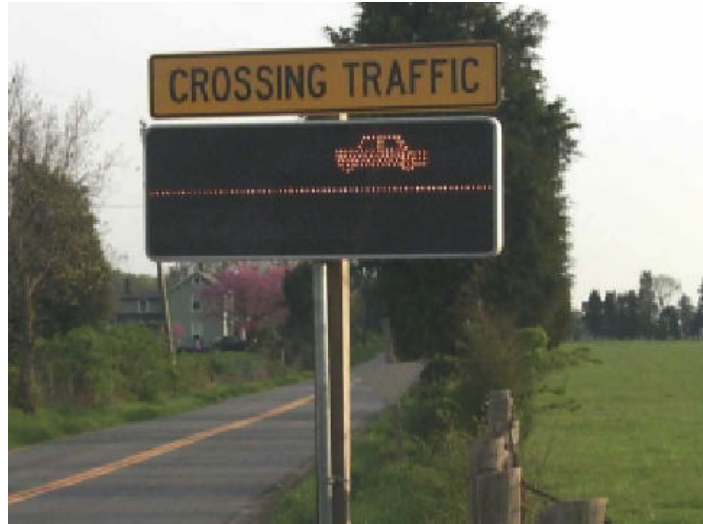
Figure 2.14. Intersection collision warning system minor approach (36)
