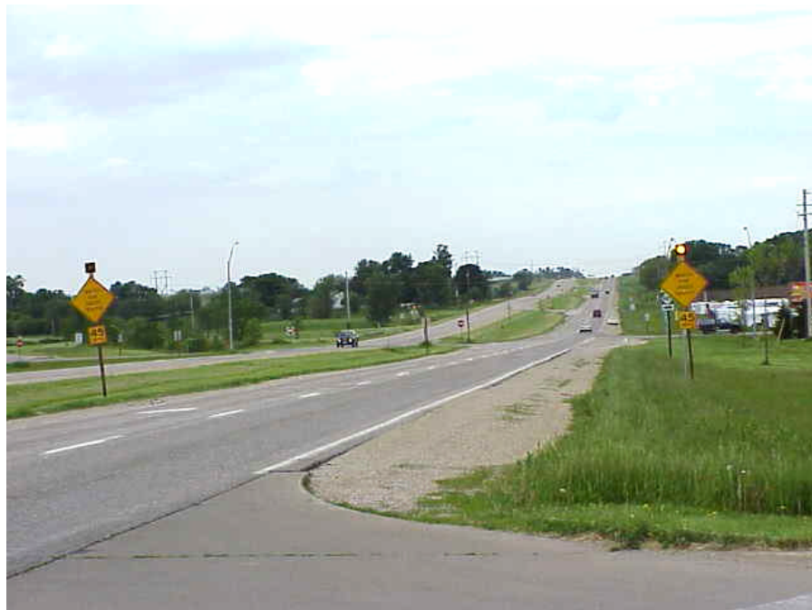
Figure 3.6. Full view of advisory speed beacon, US 65, Bondurant, Iowa
