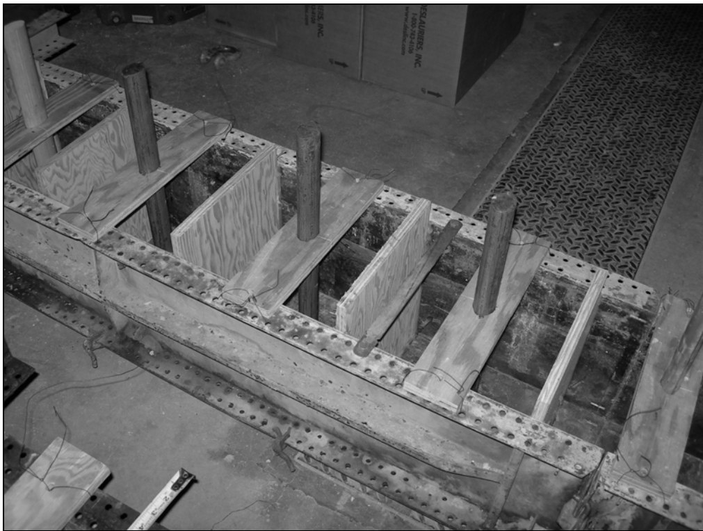
Figure 2.8. Cantilever dowel forms
