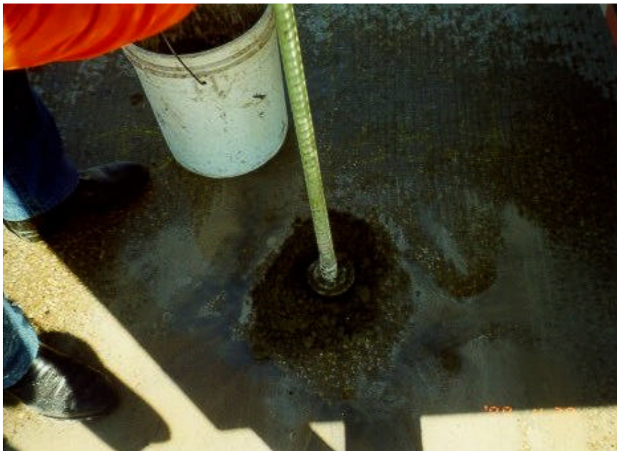
FIGURE 4.6 Patching the Cored Hole after a Core Being Extracted
