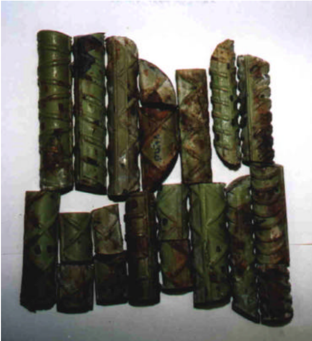
FIGURE 6.3 Rebars Samples with Significant Corrosion
