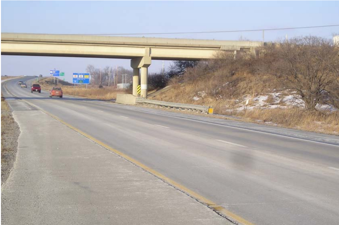
Figure I.2. W-beam guardrail and concrete retaining wall combination at outside pier
