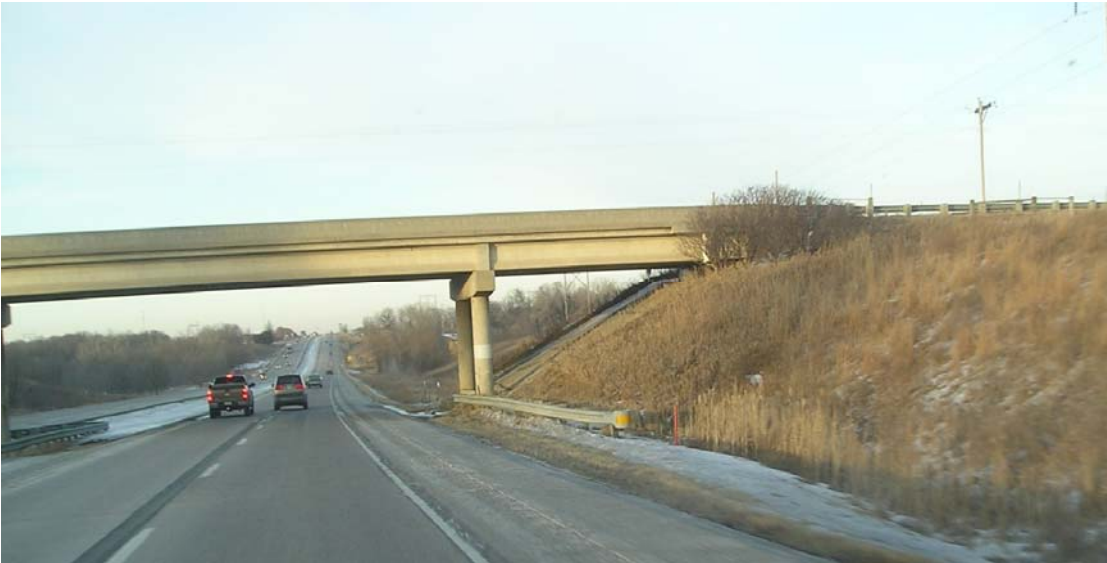
Figure I.1. W-beam guardrail at outside pier
