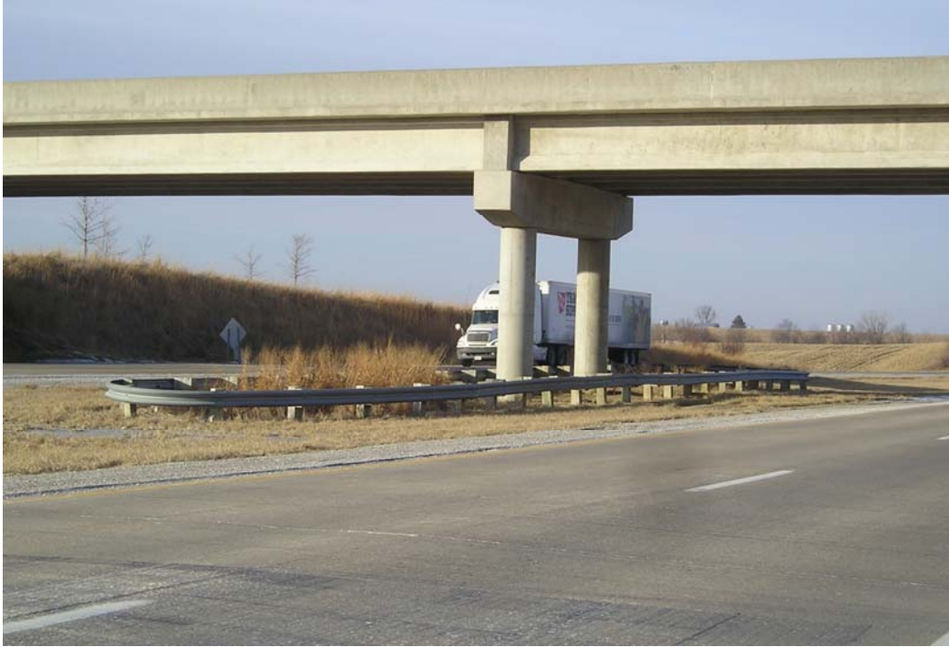
Figure I.3. W-beam guardrail in median
