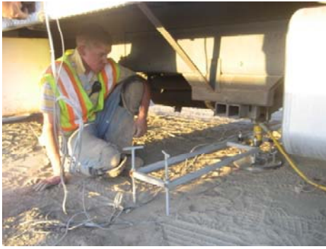
Static Plate Load Test
