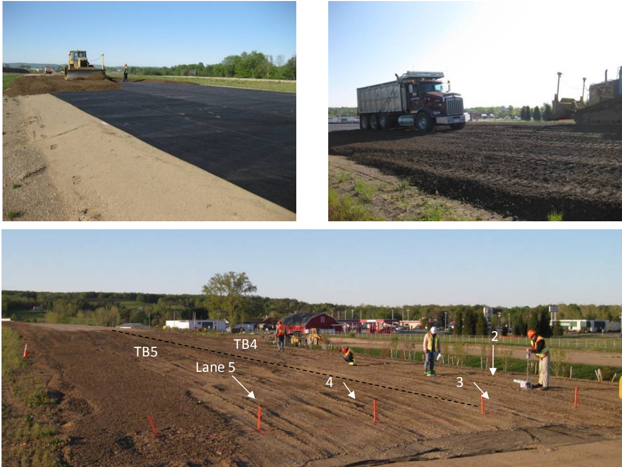
Figure 29. Construction of TBs 4 and 5 gravel subbase material calibration test strips
