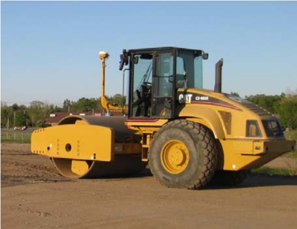
Caterpillar roller used on TB4
