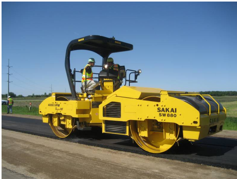
Figure 9. HMA non-wearing course layer compaction/mapping operation
