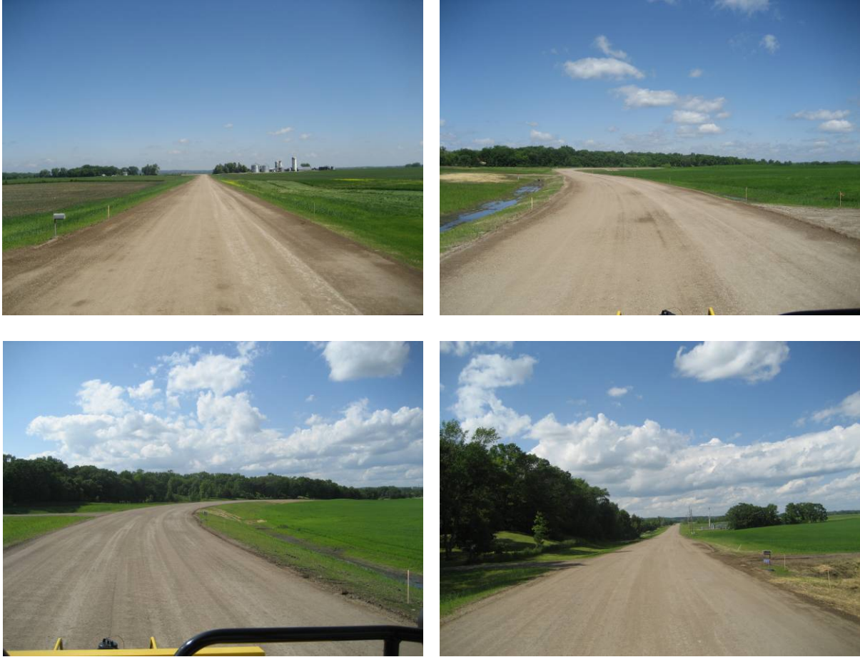
Figure 2. Photos of subbase layer along Route 4
