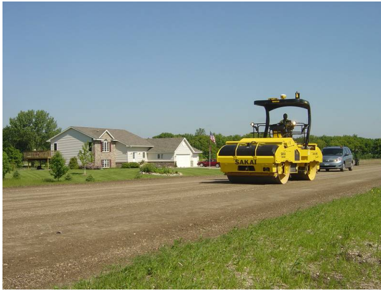
Figure 8. Subbase layer mapping operation (photo courtesy of Sakai)
