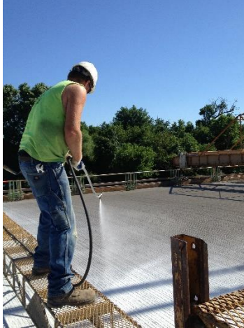
Figure 11. Curing compound being applied
