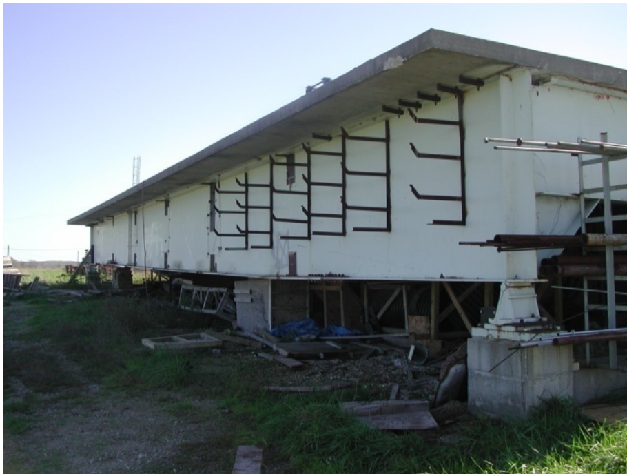
Figure 5. Full-scale bridge deck at the RTF prior to removal from site
