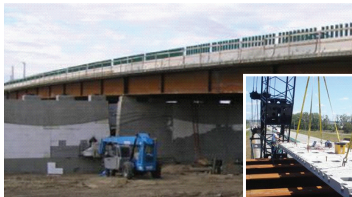
Girders on west center pier during Phase I construction
