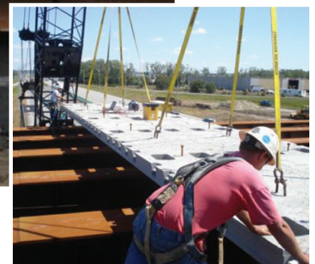
Placing precast deck panel on girders
