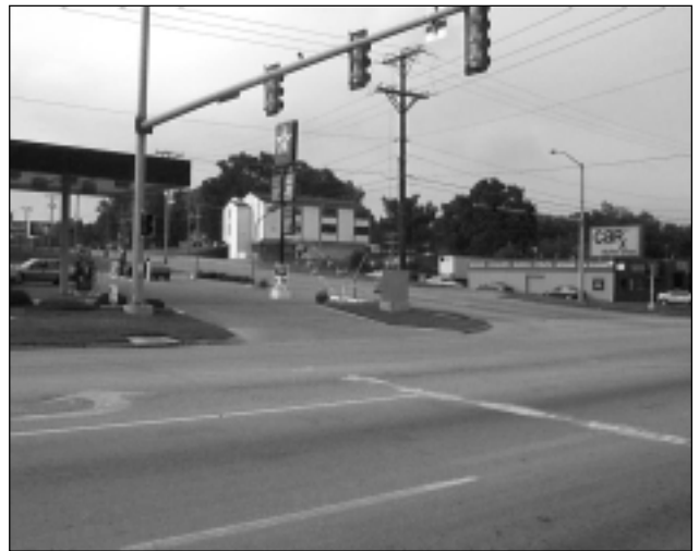
An insufficient corner clearance can create an operational and safety hazard. This intersection is ranked within the top 100 crash sites in Iowa.
