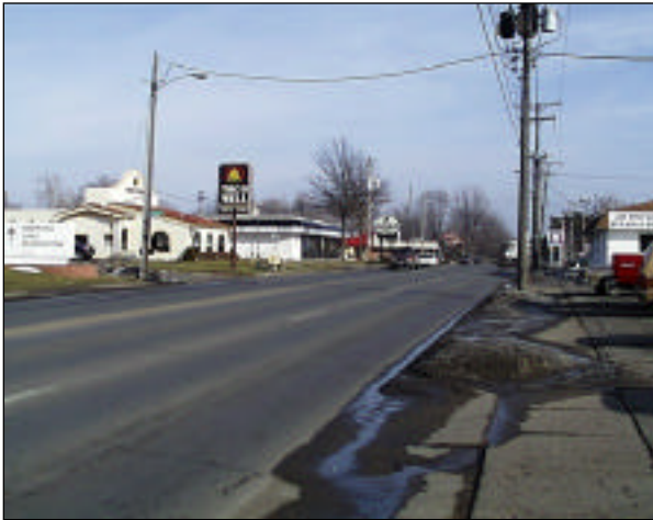
Section of unmanaged access along the Douglas Avenue/Euclid Avenue corridor in Des Moines, Iowa. Result: a high incidence of left-turn crashes.
