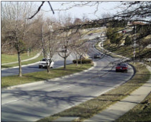
Continuous landscaped raised median on 100th Street in Clive, Iowa. Left-turn lanes are provided at intersections at widely spaced intervals.
