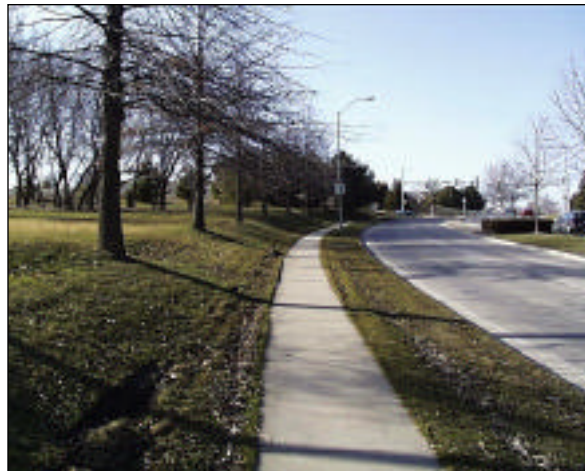
Wide clear zone with good lighting on 100th Street in Clive, Iowa. The sidewalk is well delineated, trees are located a good distance from the roadway, and utilities are underground.
