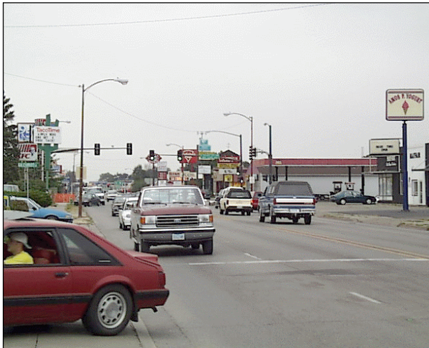
A pedestrian-unfriendly corridor: high driveway density, poor sight lines, sidewalks next to the street, and no refuge for crossing pedestrians.
