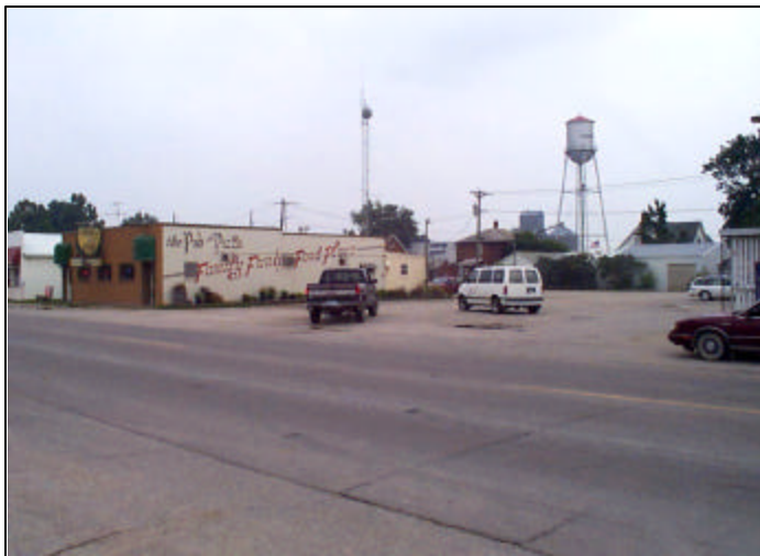
This driveway on US 218 in southeastern Iowa is too wide. It lacks curbs and discernable boundaries. This creates confusion for motorists and very unsafe conditions for pedestrians.
