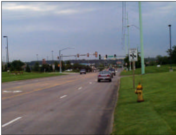
Five-lane arterial with a TWLTL, 50th Street in West Des Moines, Iowa.
