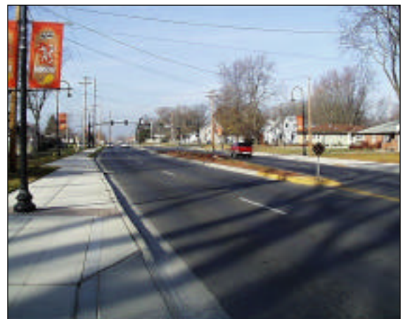
Raised median, landscaped with brick paving, at intersection of Douglas Avenue and 72d Street in Urbandale, Iowa. Adjacent land use is residential.
