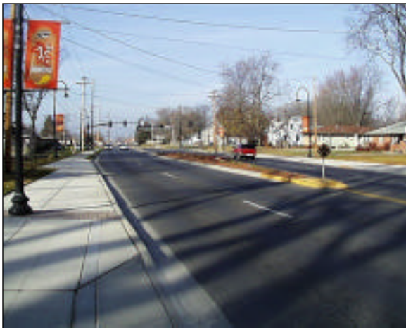
Wide clear zones on Douglas Avenue in Urbandale, Iowa. Utilities and fire hydrants have been set back a good distance from the roadway. Uniform, attractive lighting creates visual appeal.
