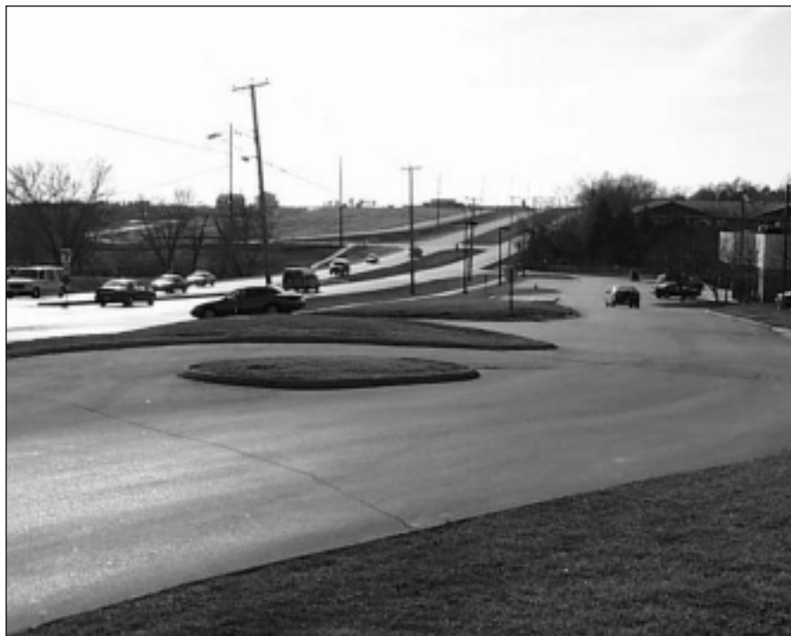
Frontage roads along Douglas Avenue in Urbandale, Iowa. The frontage road system is visible on both sides of the main roadway.
