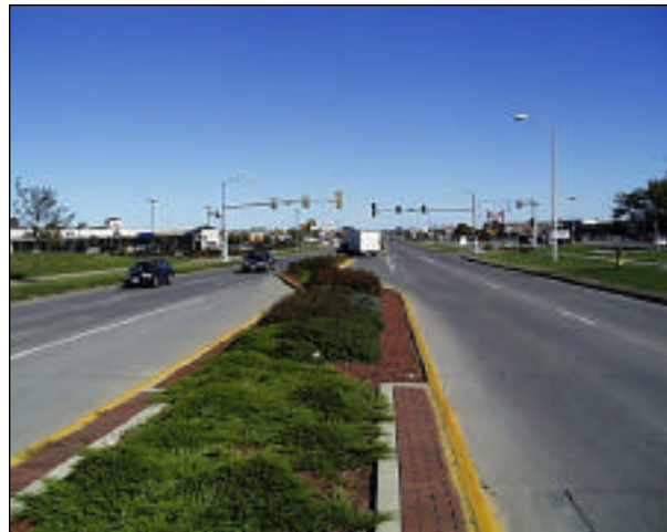
Four-lane arterial with raised median, Ankeny Boulevard, Ankeny, Iowa.
