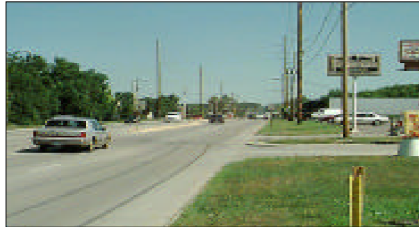
Iowa Highway 28 (1st Street/63d Street) in West Des Moines/Des Moines after retrofit with a continuous raised median, left-turn lanes at major intersections, driveway consolidation, and some widening of business driveways. Some property was purchased to accommodate a wider right-of-way.
