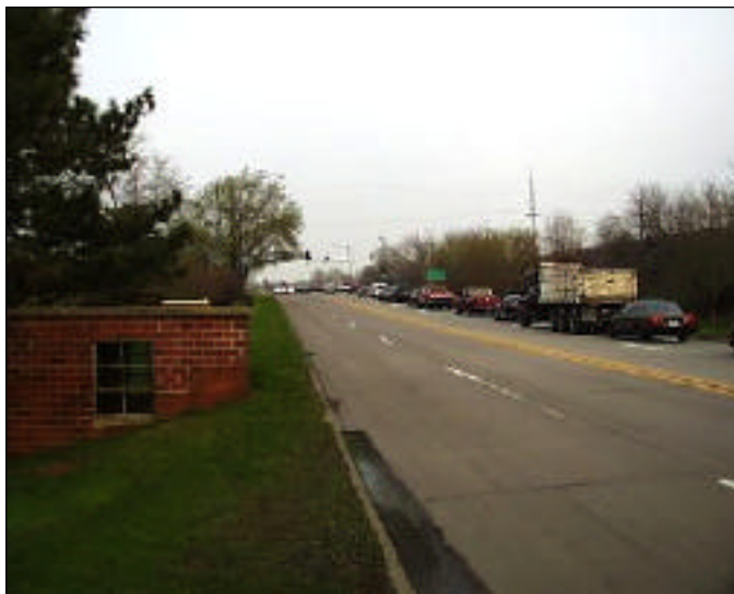
A four-lane undivided street operating as a "defacto" three-lane street. Most of the through traffic is in the outside lane, and the inside lane is used almost exclusively by turning traffic. These streets are candidates for conversion to three-lane streets.
