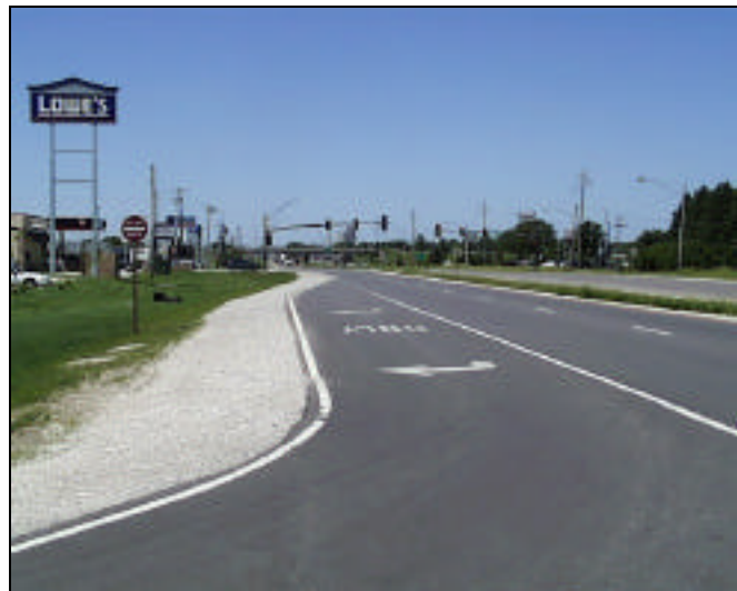
Right-turn lane at a major commercial driveway on US 69 (Duff Avenue) in Ames, Iowa.
