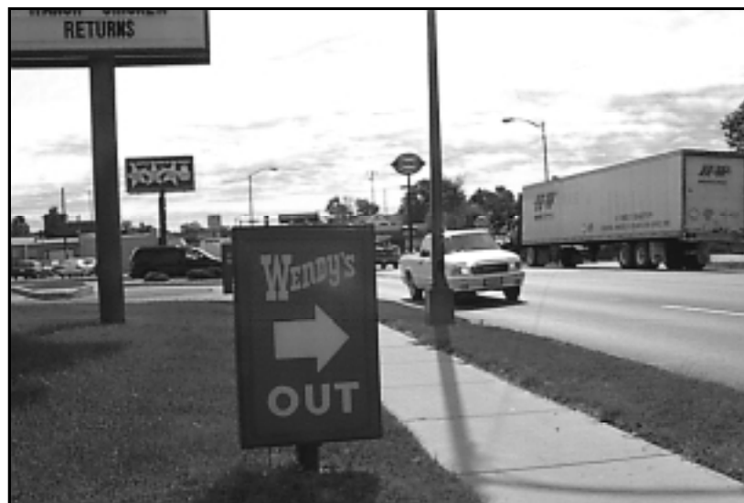
Example of inadequate sight distance as viewed from the driveway. The exiting driver cannot see far enough to safely enter the traffic stream. This situation presents an operational and safety concern.
