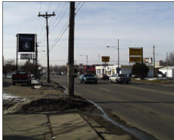
Inadequate clear zones on Douglas/Euclid Avenue in Des Moines, Iowa. Utilities are located too close to the curb. Driveways and sidewalks, which have been blocked by snow and ice, are not well delineated.
