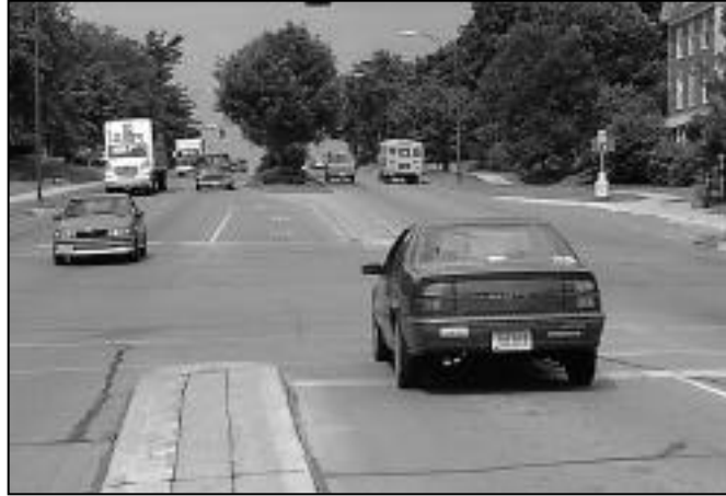
Left-turn lanes and raised medians on Lincoln Way in Ames, Iowa.
