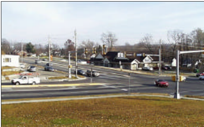
Raised median at intersection of University Avenue and 63d Street in Des Moines, Iowa. Land use at corner is primarily commercial.
