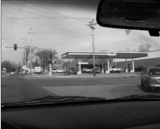
A long corner clearance at a new convenience store on University Avenue in Windsor Heights, Iowa. The first driveway is over 75 feet (five car lengths) from the corner on the left side of the picture.
