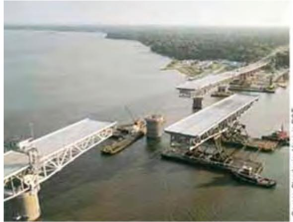
**Figure 17. Barges floating a prefabricated segment to installation location**
