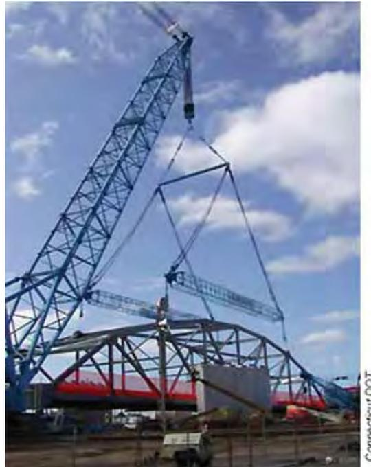
**Figure 16. Placement of a prefabricated steel truss on Church Street Bridge**
