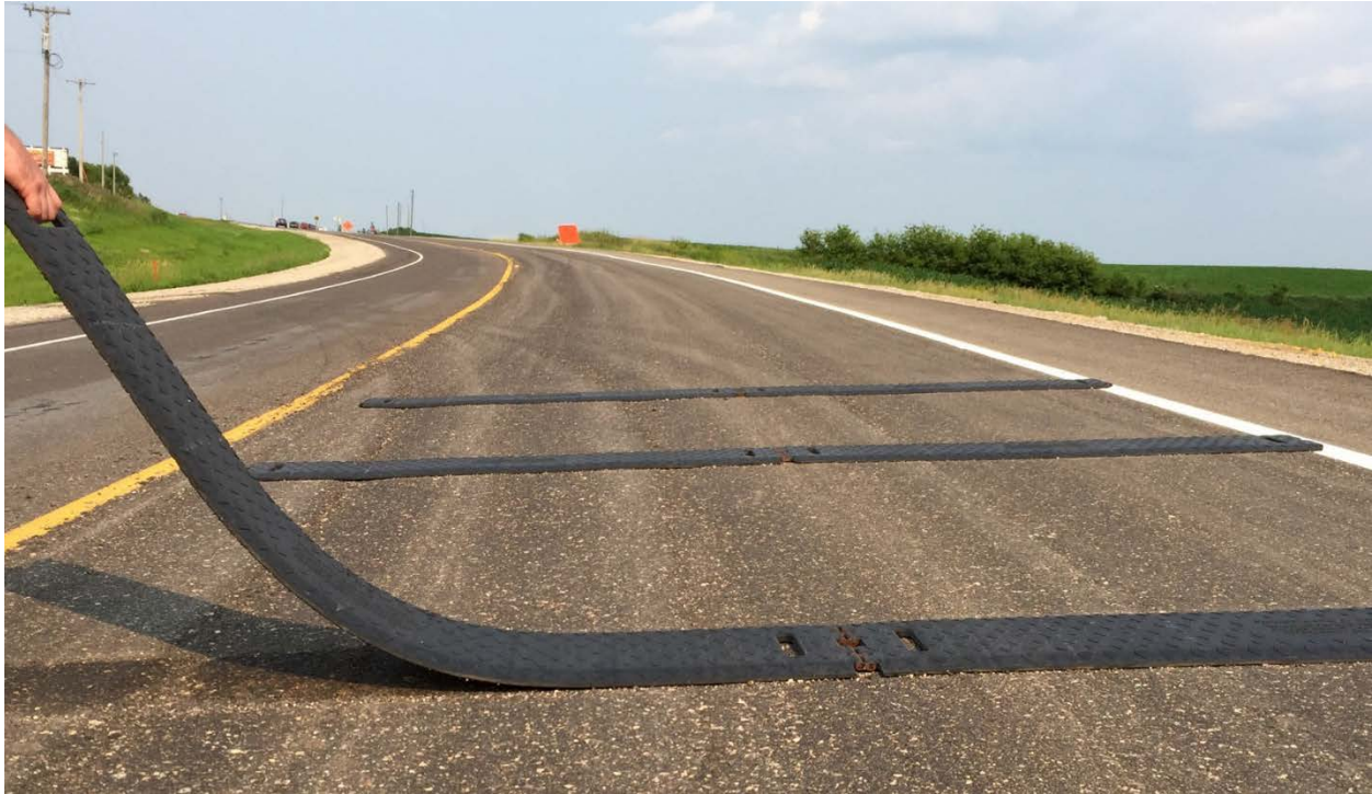
Figure 1. Temporary rumble strips
