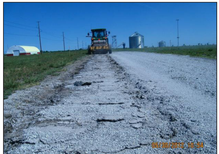
Figure 2. Chip seal coat surface during high-energy IR (HEIR) compaction
