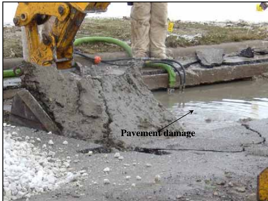
Figure 36. Saturated material being excavated
