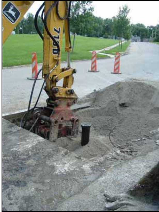
Figure 41. Backfill compacted into trench
