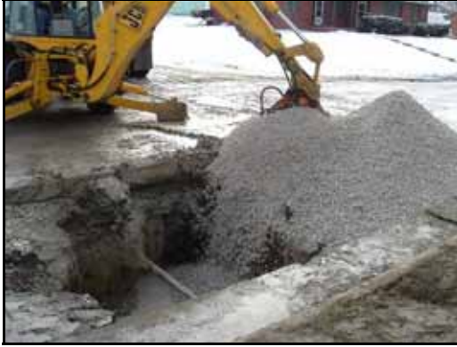
(a) Pushing in backfill material
