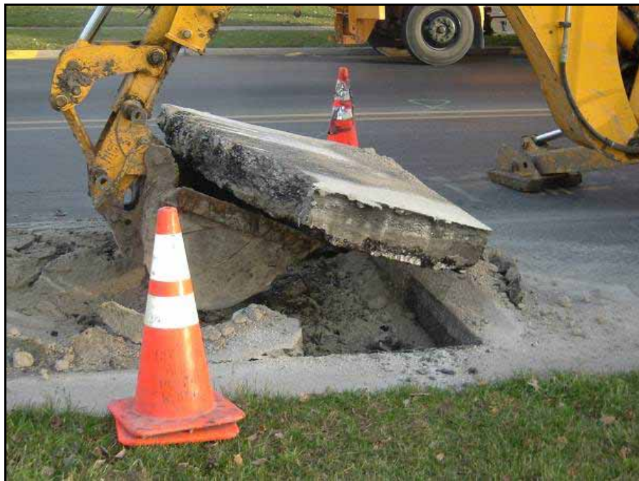
Figure 31. Pavement removal
