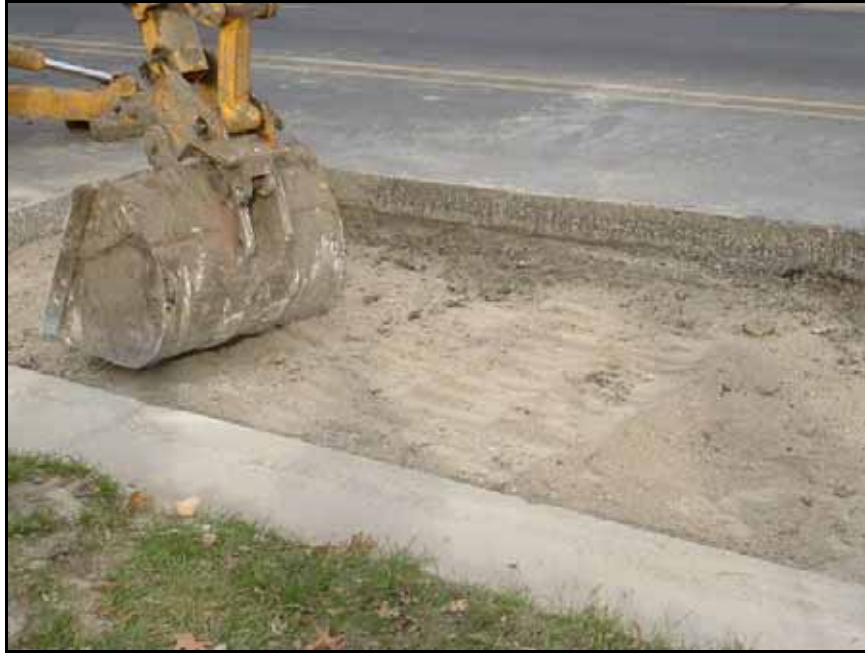
Figure 32. Backhoe bucket compaction
