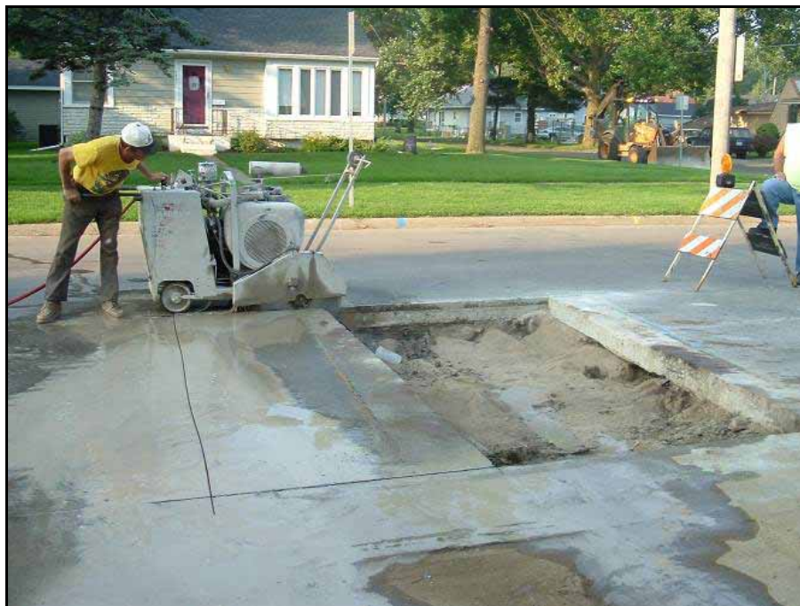
Figure 46. Concrete pavement cut being made
