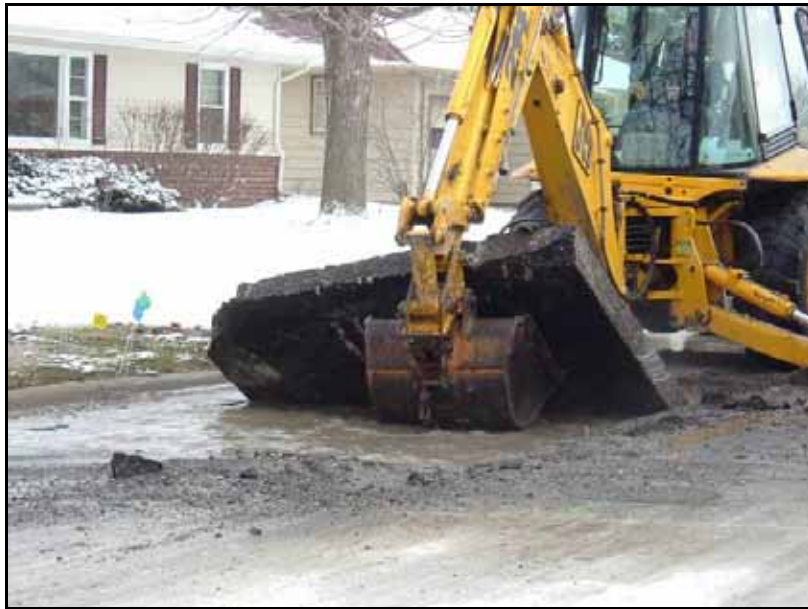
Figure 34. Pavement removal from Ames winter break site
