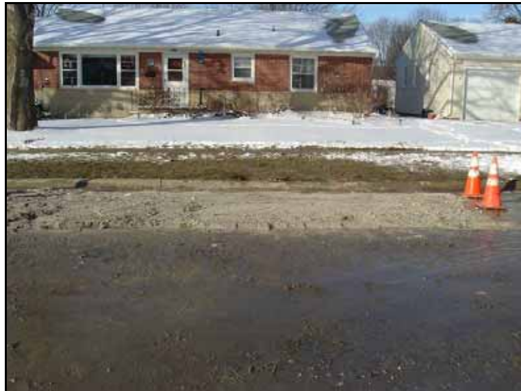
Figure 39. Trench ready for cold patch
