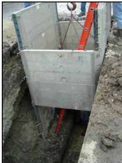
Figure 26. Shoring box placed into trench
