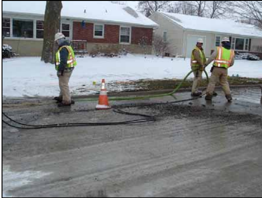
Figure 35. Dewatering the trench
