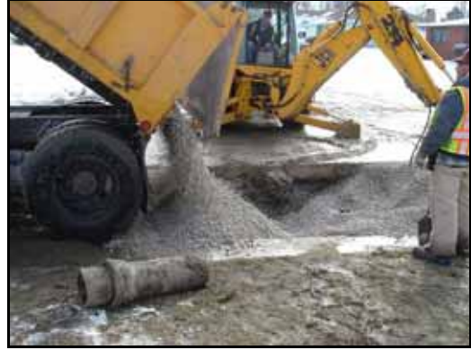
(b) Dumping backfill material
