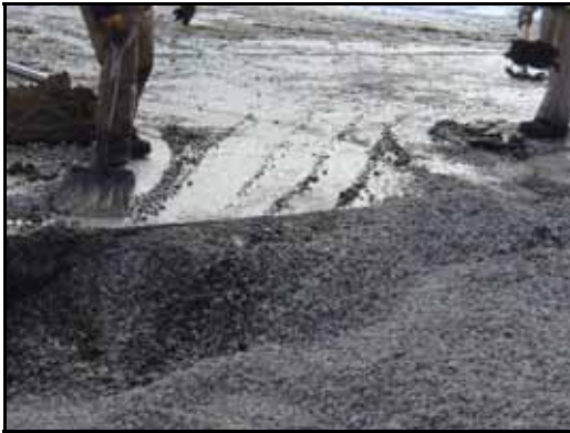
(a) Cleaning excess material into the trench
