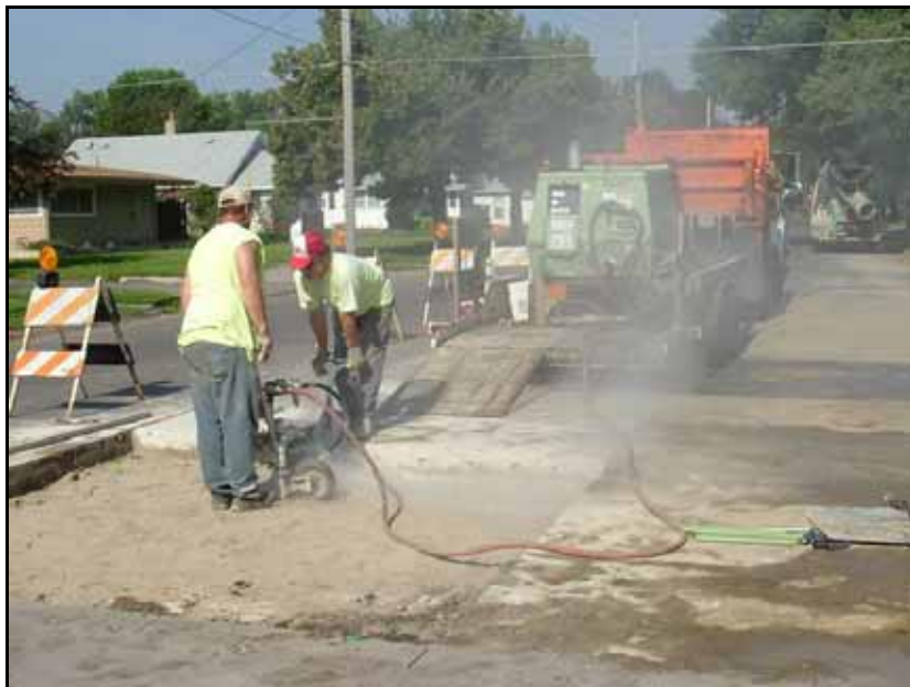
Figure 48. Drilling spacings for dowel bars
