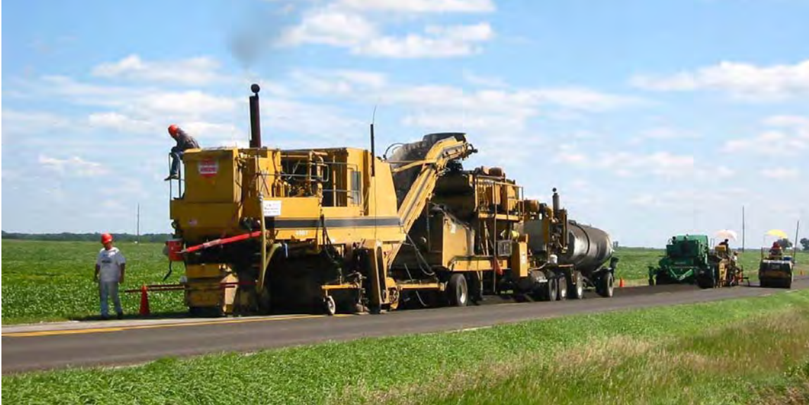
Figure 2. Picture of a typical CIR recycling train
