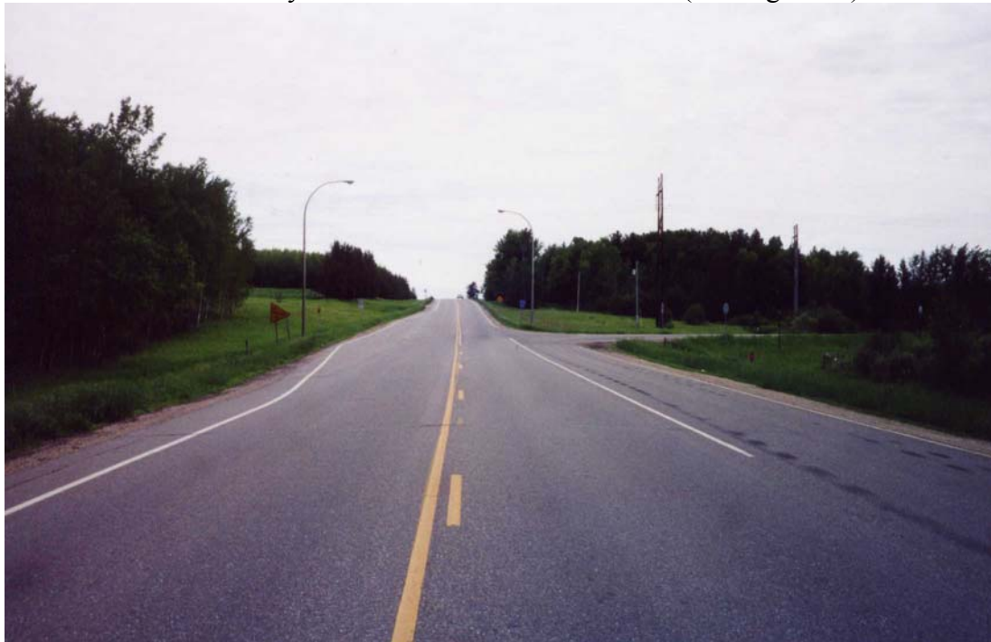
Cass County: TH 64 and CSAH 33 (looking south)
