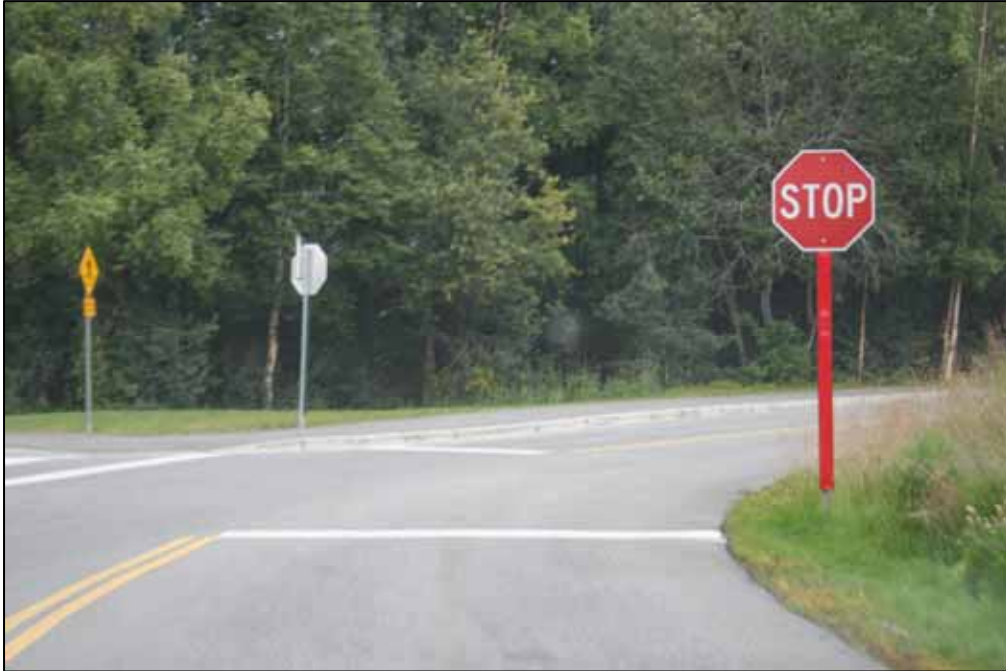
Figure 5. Reflective strips on stop sign (Image source: Neal Hawkins)
