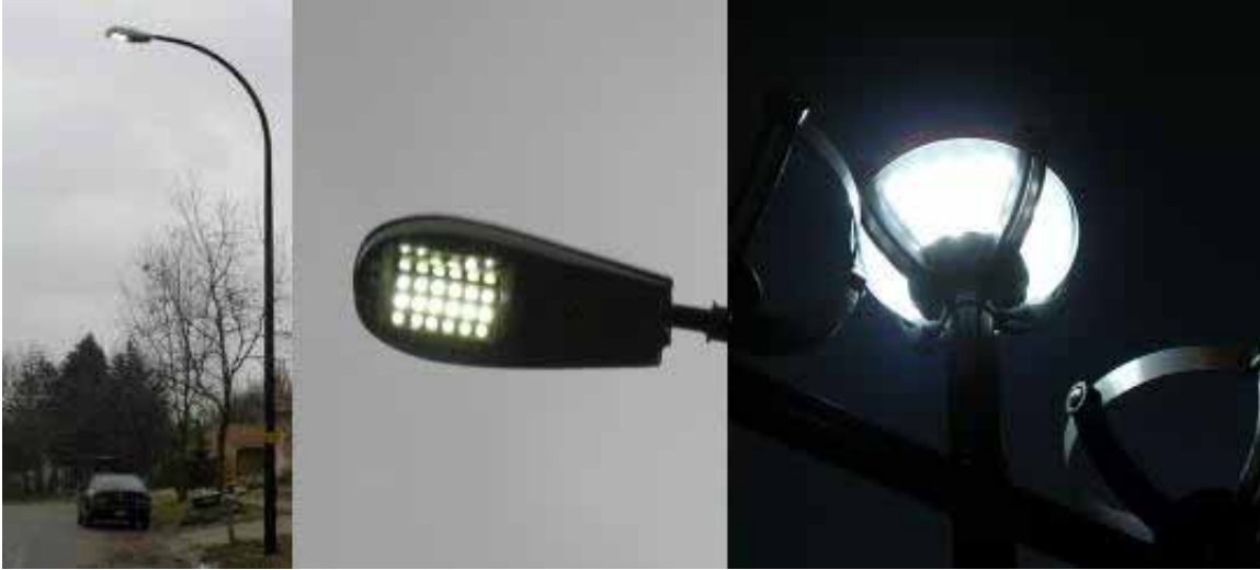
Figure 5-6: Cobra head (left and center) and globe LED lights evaluated in Ann Arbor (Image source: City of Ann Arbor, 2007)
