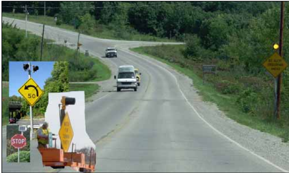
Figure 3. Flashing beacons in a variety of settings (Image source for LED Stop Sign: TAPCO, all other images Neal Hawkins)
