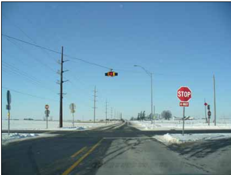
Figure 9. Use of overhead flashing beacons at all-way stop intersections (Image source: Neal Hawkins)
