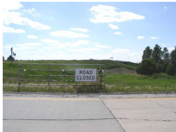
Figure 4.2. Left-side swing gate on entrance to I-35
