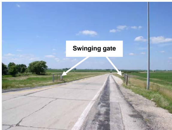
Figure 4.1. Gates on entrance ramp to I-35
