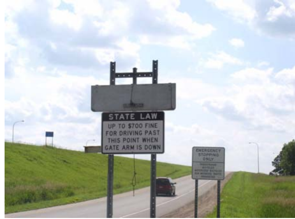
Figure 1.4. Minnesota flip-down ramp closure sign
