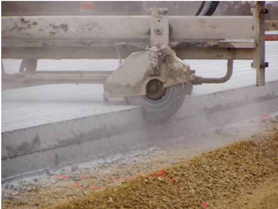
Figure A10. Transverse sawcut operations
