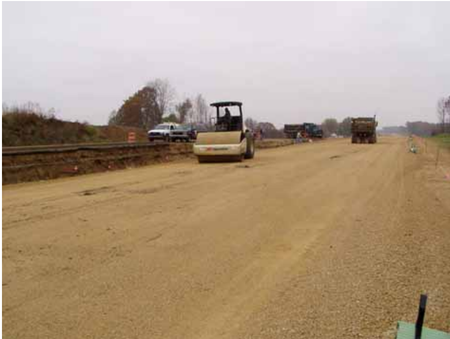
Figure A1. Base preparation and concrete delivery operations
