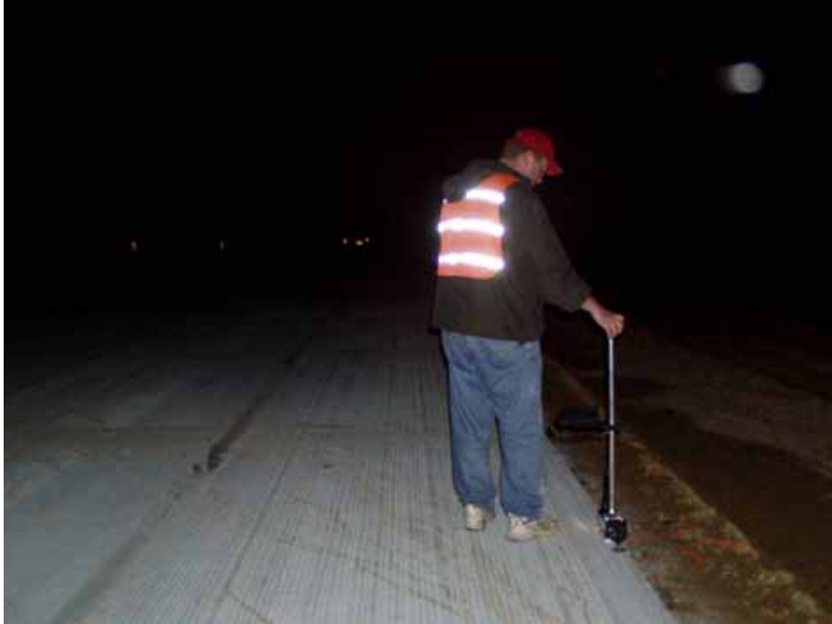
Figure A13. Inclinometer profiling
