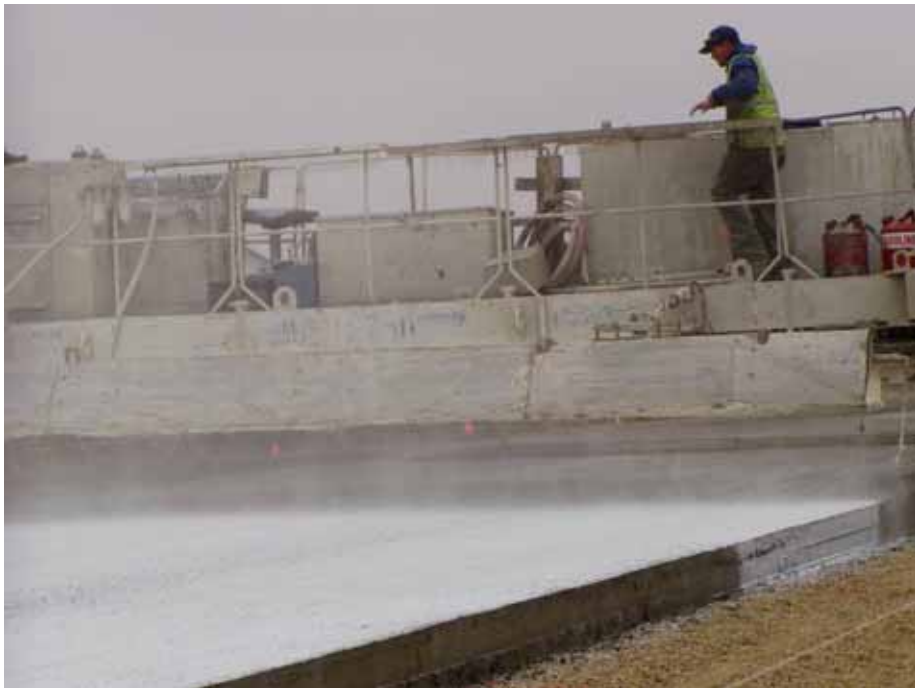
Figure A8. Curing operations
