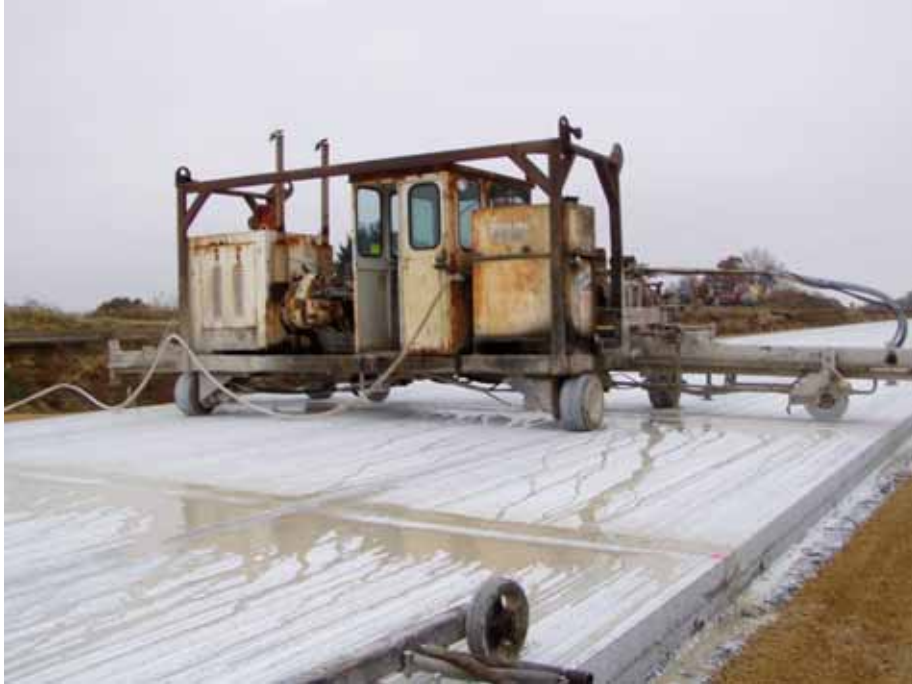
Figure A9. Transverse sawcut operations
