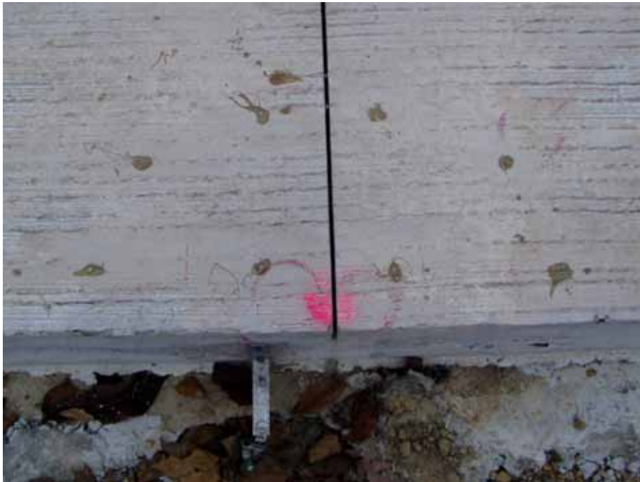
Figure A22. Corner DEMEC installation
