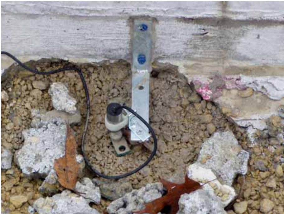
Figure A20. LVDT installation (Transtec)
