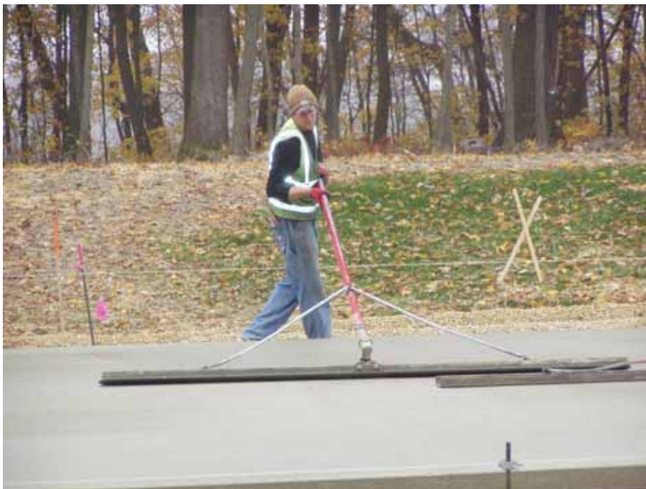
Figure A6. Straightedge operations
