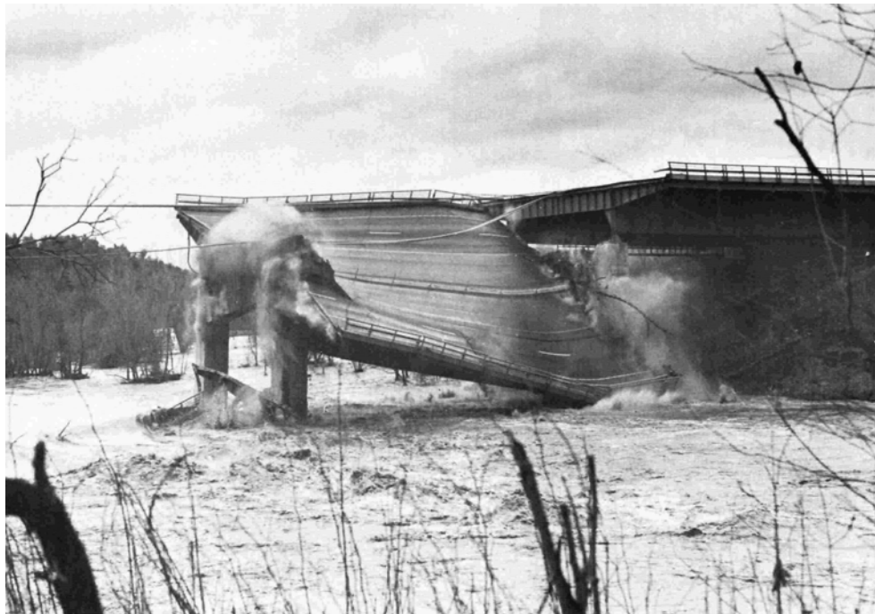
Figure 2.1. Photograph of the Skoharie Creek Bridge collapse, 1987
