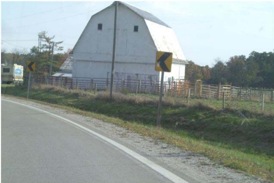
Figure A.6. County Road X-23, closer view of chevrons
