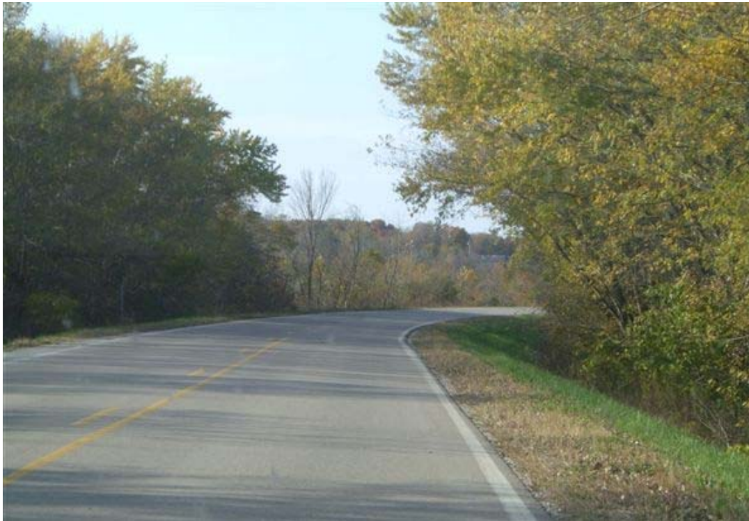
Figure A.10. County Road W-62, close proximity of vegetation along horizontal curve
