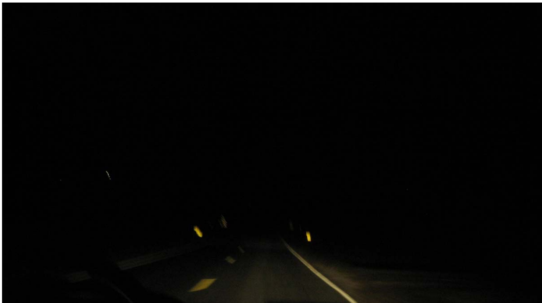
Figure A.8. Nighttime view of pavement markings and guardrail delineation at bridge
