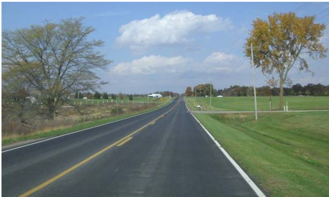
Figure A.2. Pavement markings on County Road H-46
