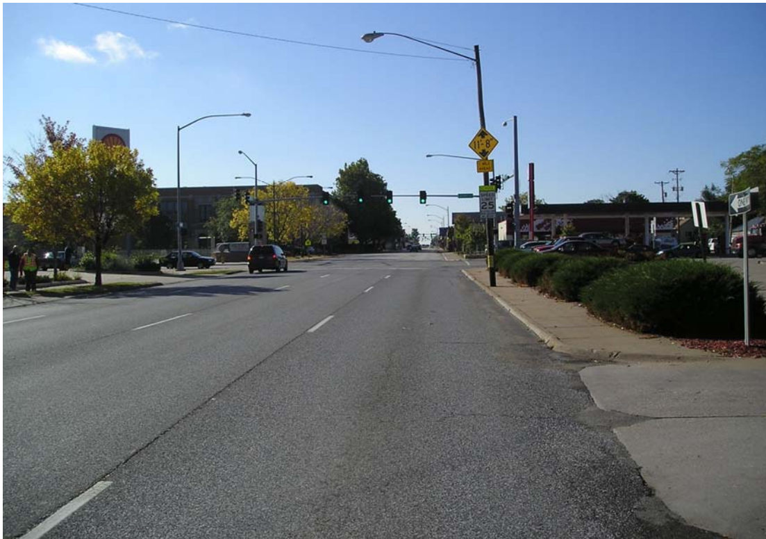
Figure A.6. Southbound Harrison Street
