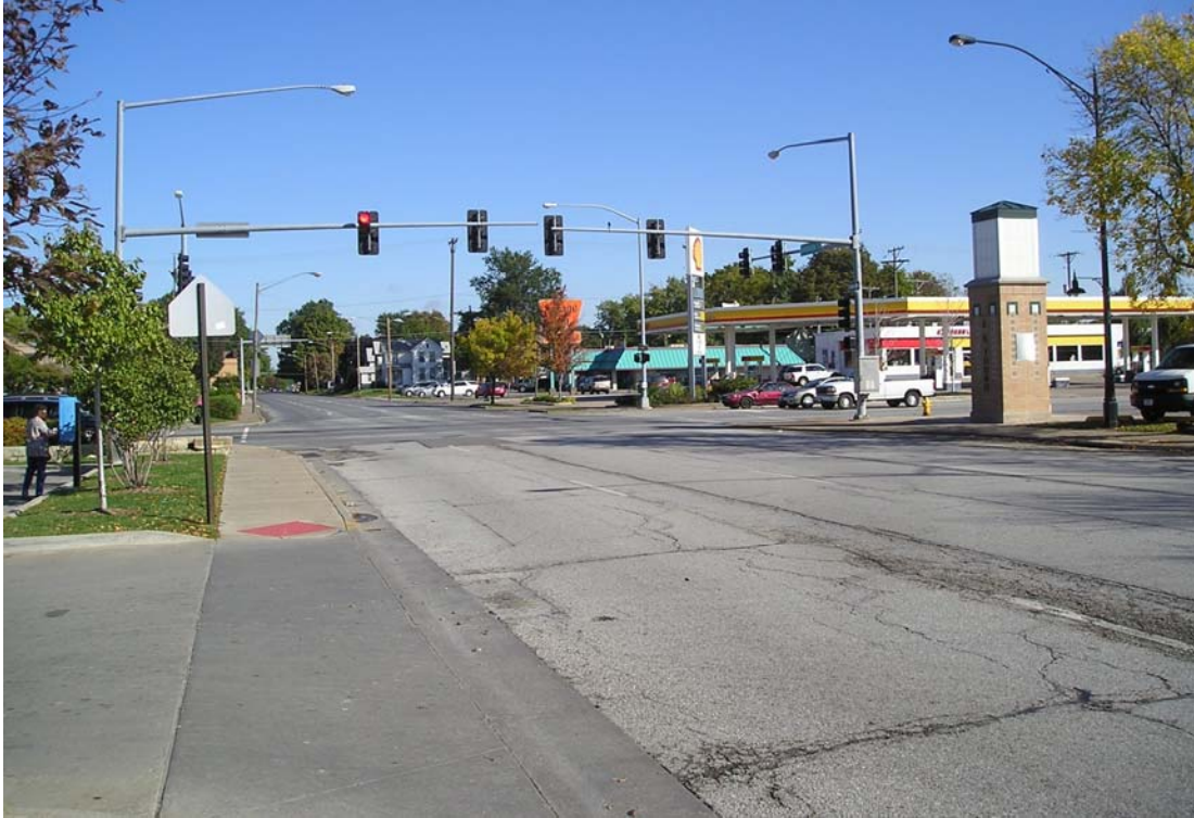
Figure A.7. Tattle-tail signal for southbound Harrison Street traffic
