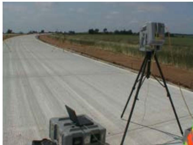
Figure 9. Highway 5 (New Concrete Pavement)
