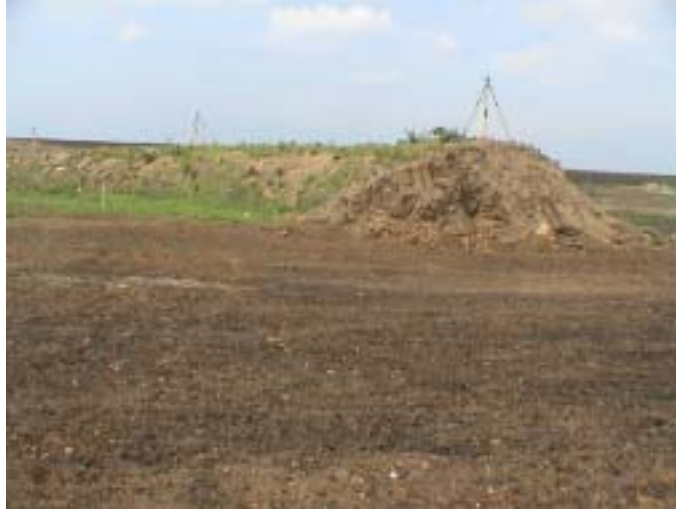
Figure 14. Side View of Stockpile
