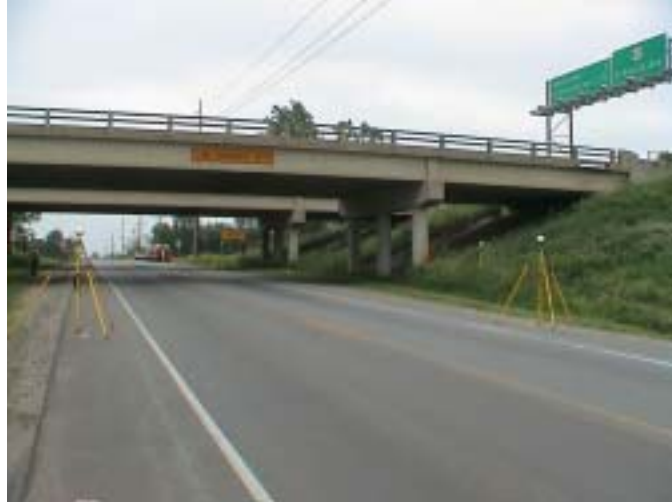
Figure 8. Southbound Broadway Bridge (Pair of Bridges)
