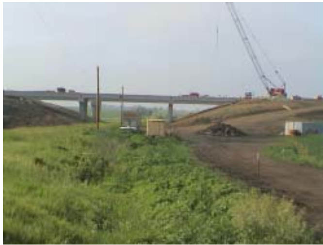
Figure 10. Hardin County Bridge Facing South (Bridge Beams)
