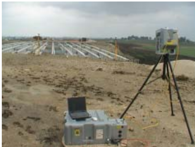
Figure 11. Hardin County Bridge Facing East (Bridge Beams)
