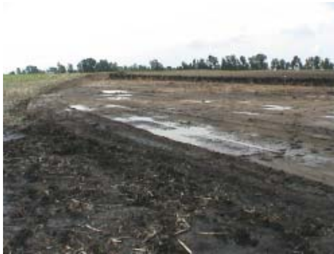
Figure 15. I-35/I-80 Borrow Pit
