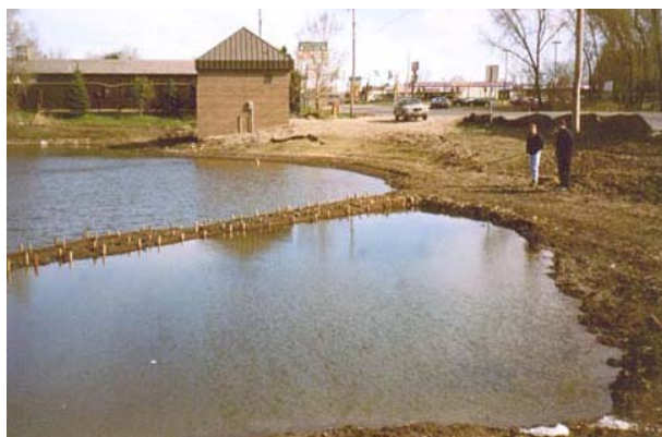
Tanners Lake alum injection facility - Oakdale, MN Source: Minnesota Stormwater Manual
