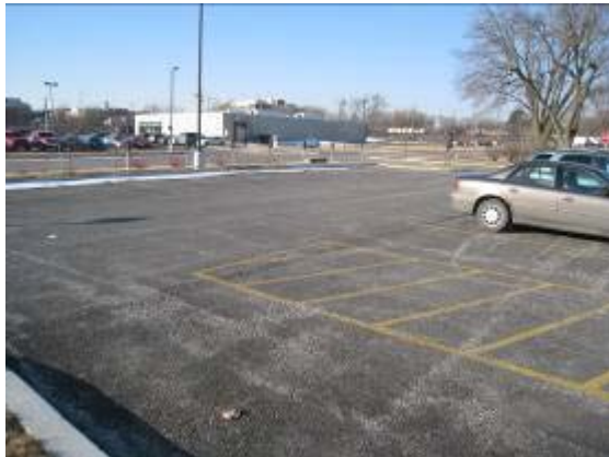
Porous Asphalt Parking (Lot 121 – Iowa State University)
