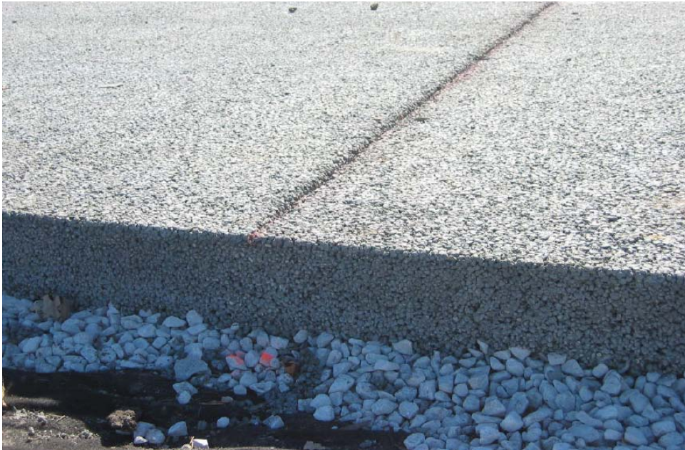
Figure 7: Pervious concrete surface and conventional PCC (Iowa State University Lot 122)
