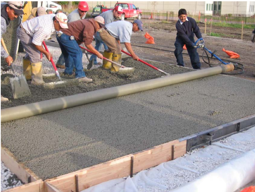
Figure 10: Roller screed finish operation on pervious concrete material (ISU Lot 122, 2006)
