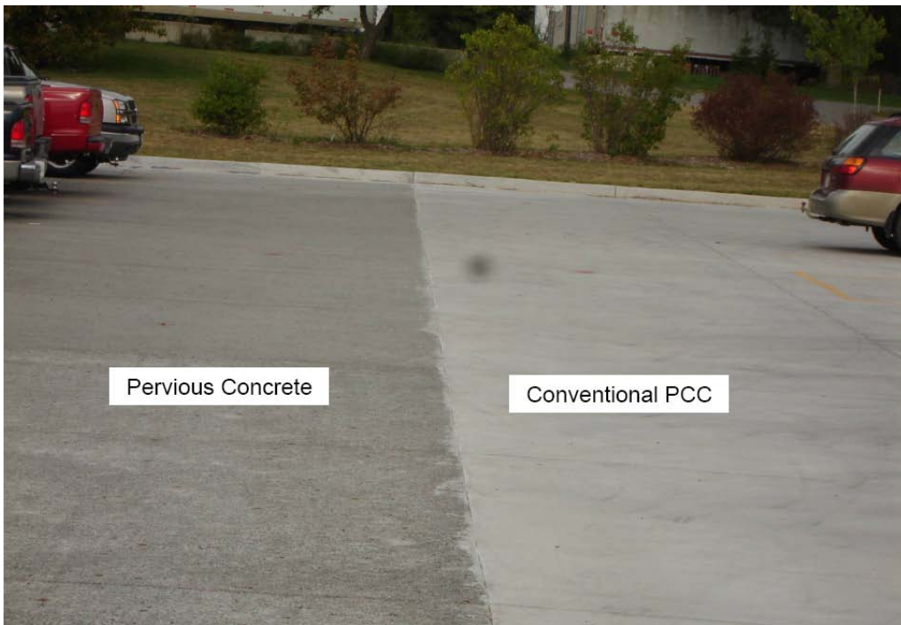
Figure 7: Pervious concrete surface and conventional PCC (Iowa State University Lot 122)
