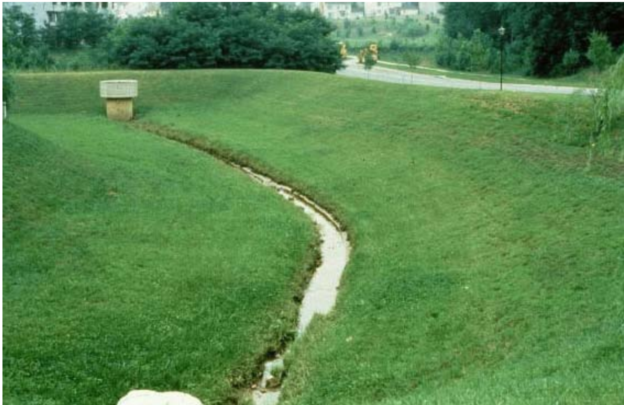
Figure 1: Dry detention basin
