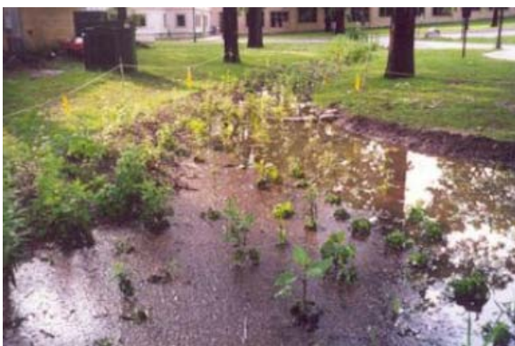
(c) Newly planted bioretention area after storm
