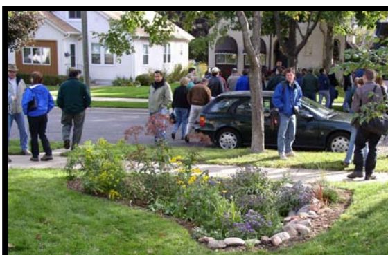
(a) Rain garden for single family residence
