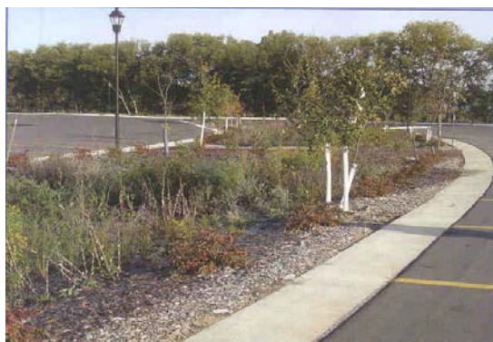
(b) Bioretention in landscaped parking lot median
