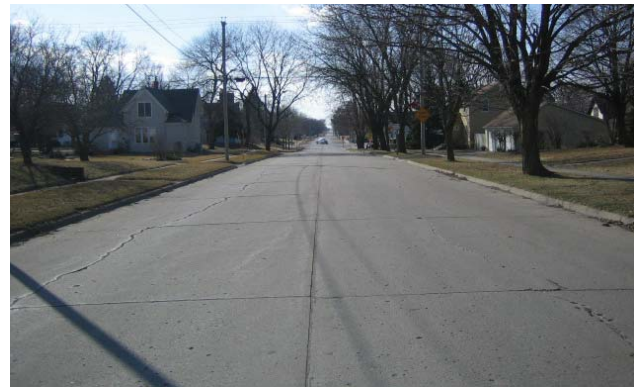
E-18 before implementation of traffic-calming treatments
