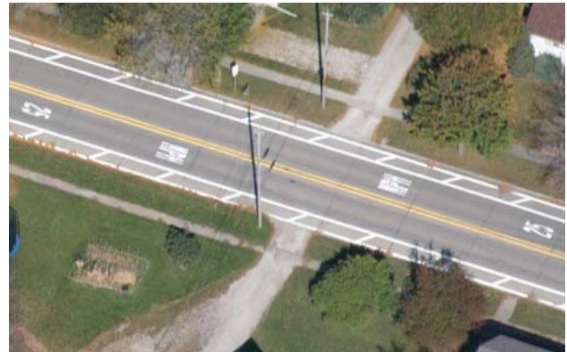
On-pavement "25 mph" speed markings and lane narrowing using painted shoulders
