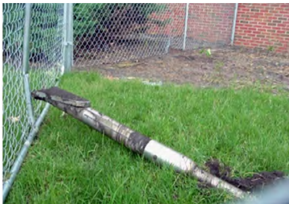
Five-inch-diameter drill bit emerging from the ground
