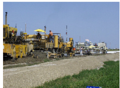
Stringless paving train
