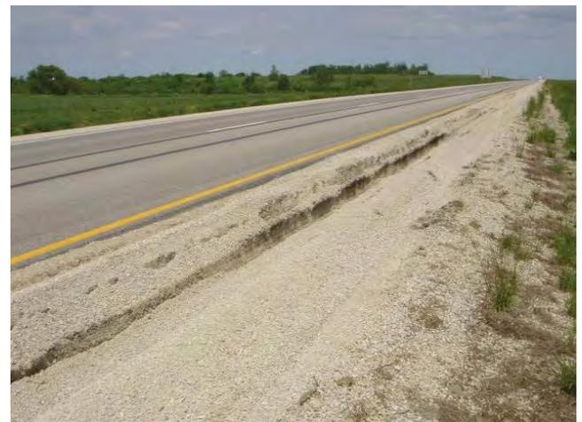
*Severe shoulder rutting caused by bearing capacity failure of the soft underlying subgrade*
