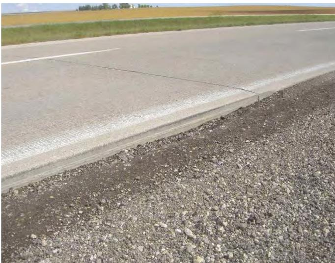
*Edge drop-off along the outside shoulder caused by vehicle off-tracking*
