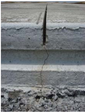
Test section joints showing different sawing depths: conventional sawing to one-third pavement thickness (left), conventional sawing to one-quarter pavement thickness (middle), early entry sawing (right)
