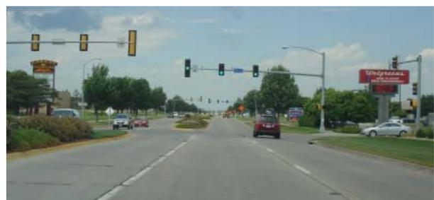
Left-turn lanes installed on a corridor in Ankeny, Iowa
