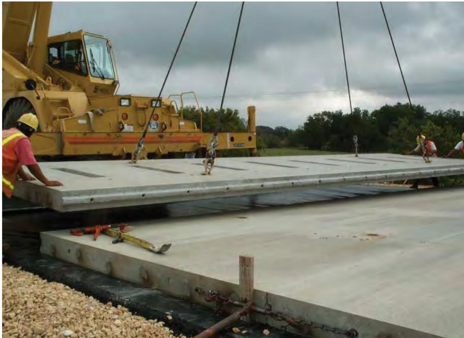
*Prefabricated concrete panel installation (photo courtesy of Dave K. Merritt, The Transtec Group, Inc.)*
