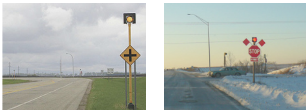
Figure 1. Sign-mounted beacons used to replace overhead flashing beacons (Image source: Mn/DOT 2006)
