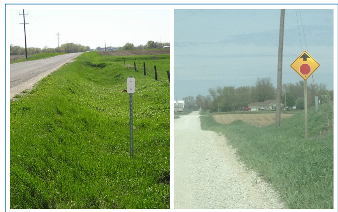
Sample Mitigation: New, highly-reflective delineators and signs installed in Dallas and Story counties
