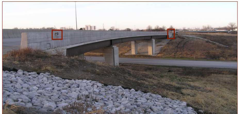
GPS antenna locations on Bridge 0309 with south abutment, left, and north abutment, right
