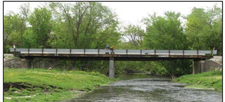
*Multiple span RRFC bridge constructed using 89-foot railroad flatcars*
