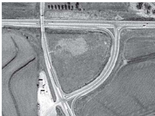
Figure 8. Intersection of US 59 and US 34 in Mills County, IA
