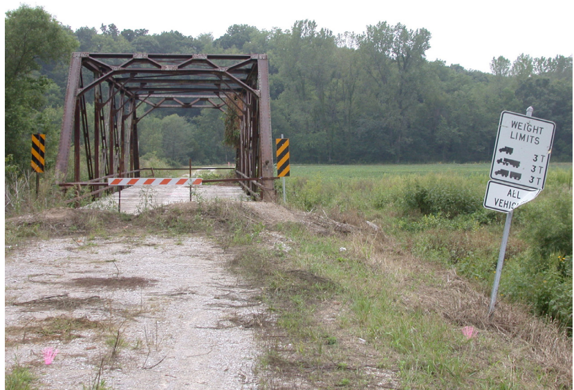
Wapello County truss bridge prior to replacement
