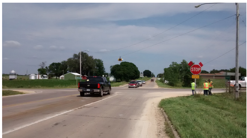
Field reviews of two two-way stop-controlled intersections, one of which also has an overhead flashing beacon, during previous RSAs in Iowa
