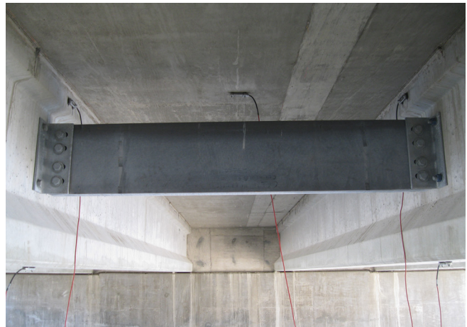
Strain gauges attached to the underside of the bridge
