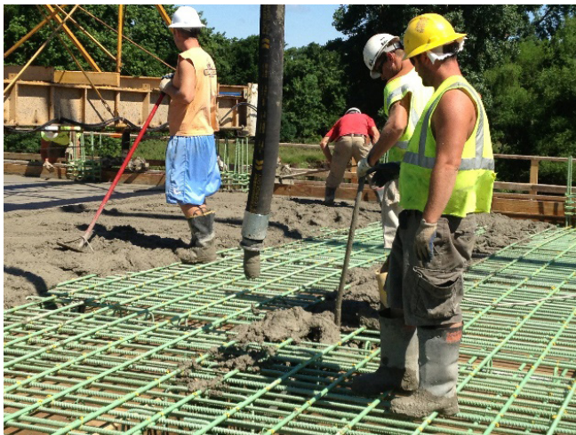
LWFA concrete placement on the bridge deck
